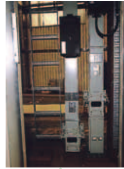
带有终端头的抬升网电源 rising mains with tap-off
