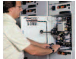
抽屉式安装方式 Withdrawable type installation
