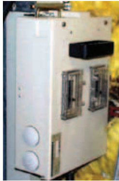
可以在带电的情况下插拔终端头 Tap-offs are pluggable under voltage
