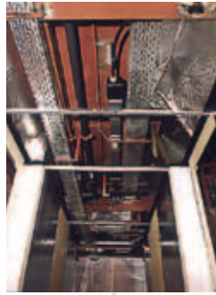
为船舱供电的地面水平母排 horizontal busbars in a floor in order to feed the cabins
